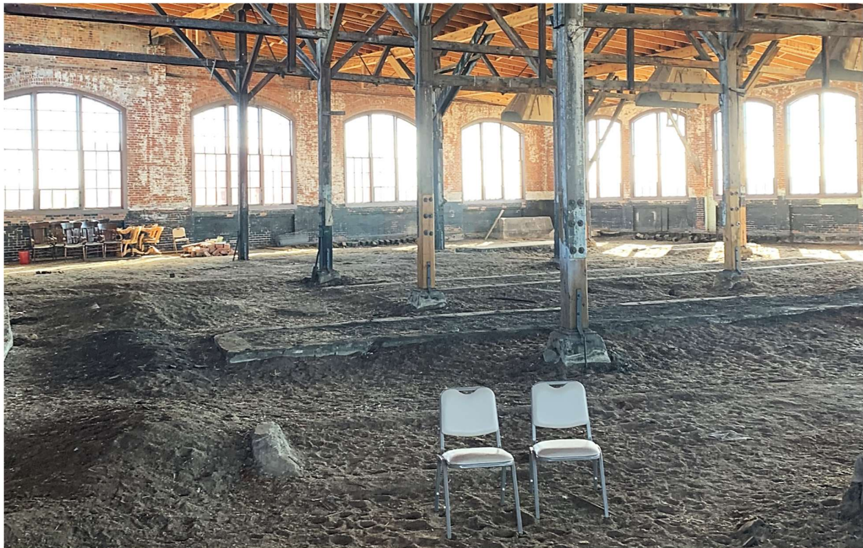
Image 5: Engine Service Pits – Upper Portion of the Concrete Stem Walls Visible
